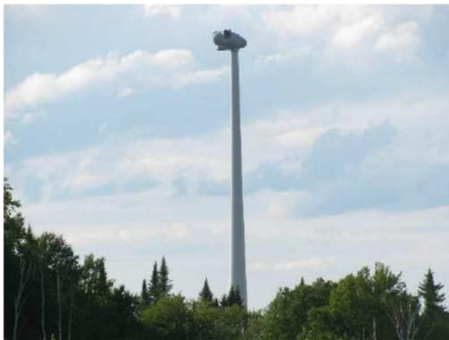
98m Wind Tower and 2 MW Nacelle Erected at New Richmond (66 MW), Quebec
