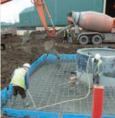
Installation of the wind turbine foundation.
